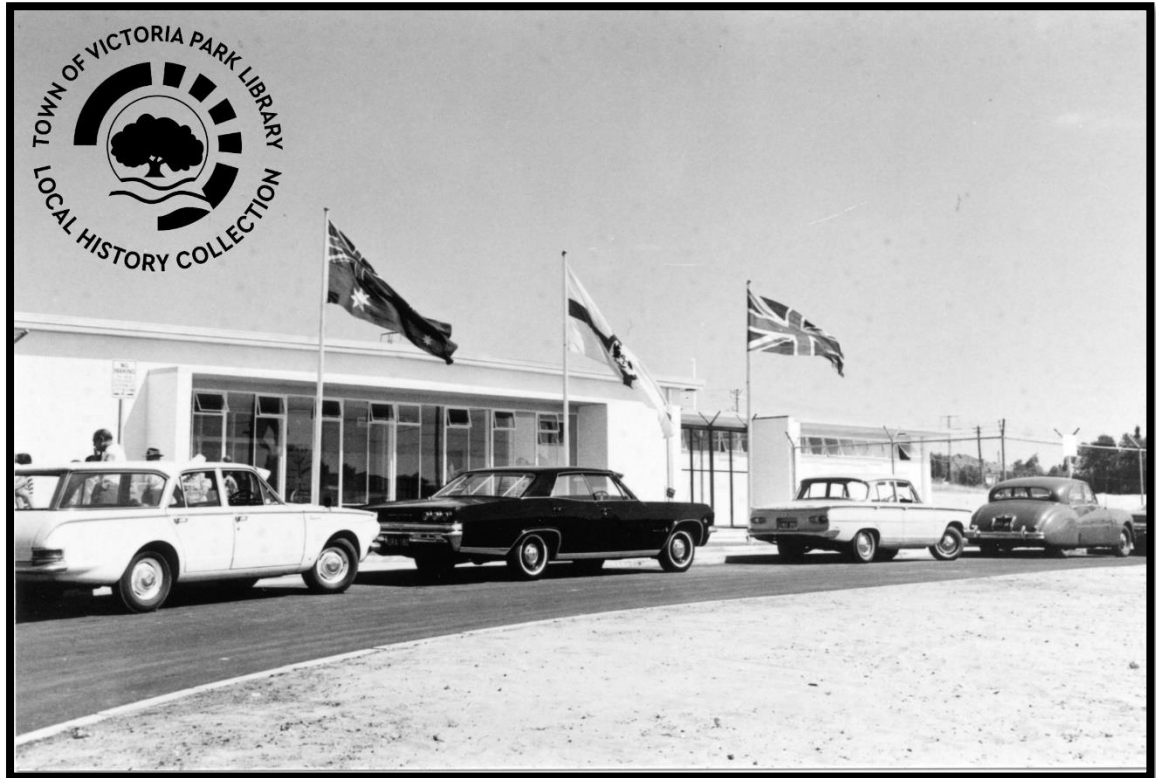
PH00233-01 Front entrance to the Somerset Pool on the day of the Official Opening, 1966. Local History Collection, Town of Victoria Park Library.
