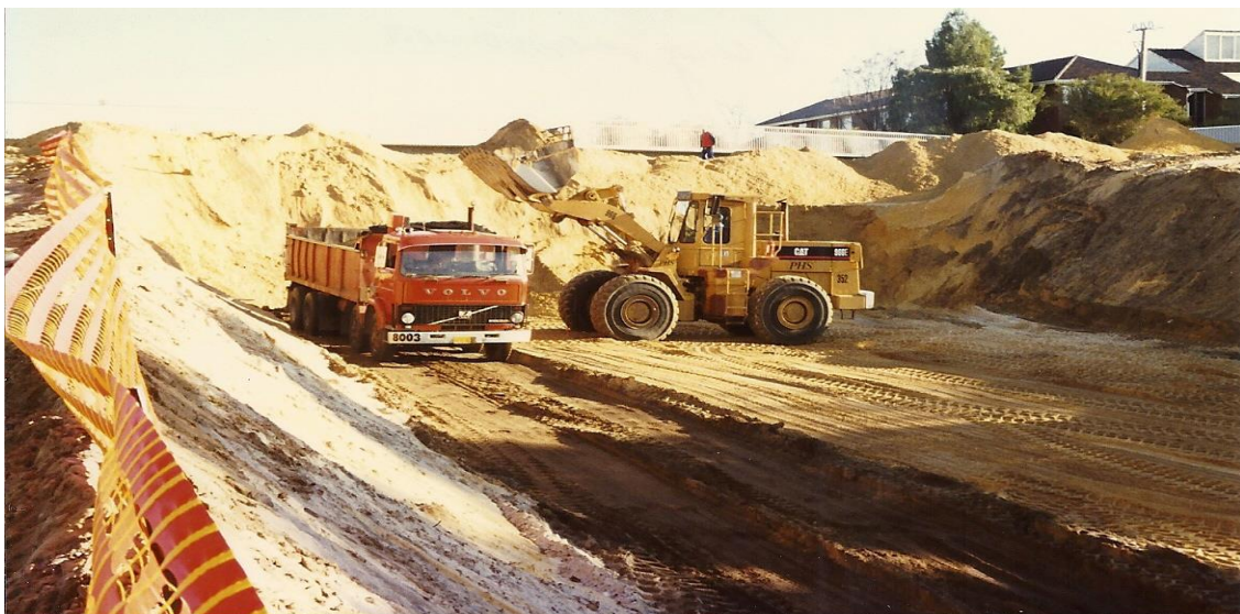
Taken from Orrong Road near the intersection of Cornwall Street showing the mountain of sand yet to be removed after the pedestrian bridge has been completed and the soil utilised on the abutment of the bridge over the highway.
