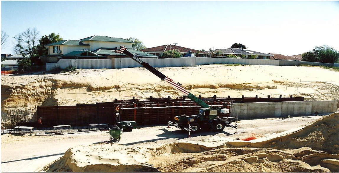
Building the concrete retaining walls through the cutting near the pedestrian footbridge.
