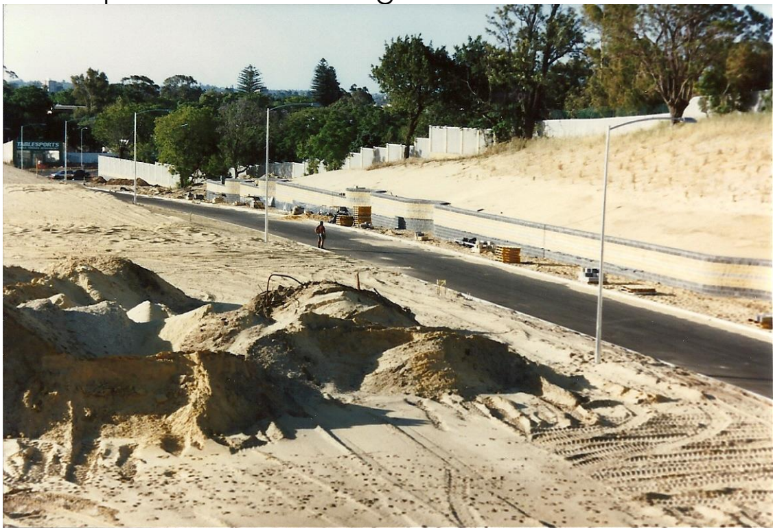
Building the concrete retaining walls through the cutting near the pedestrian footbridge.
