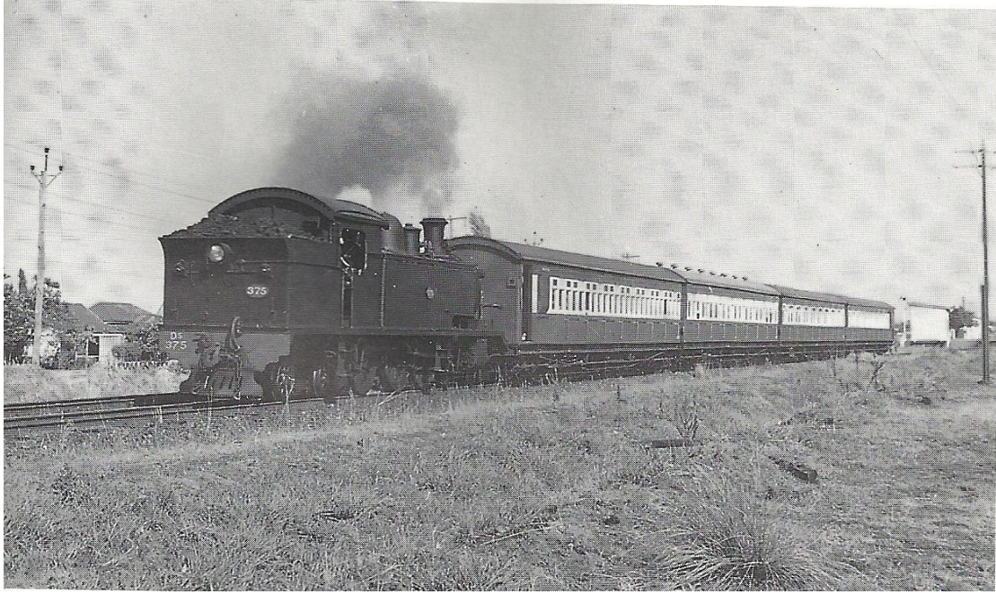
Typical Suburban Train Side Loading Doors Photo Rail Museum, Ashfield.
