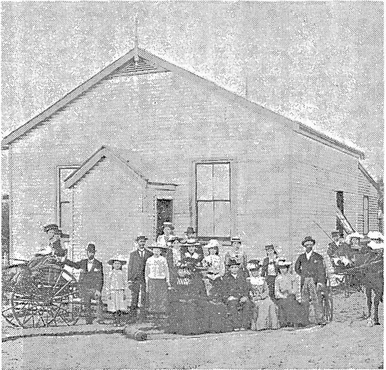
Methodist Church Albany Road 1896 Courtesy Uniting Church
