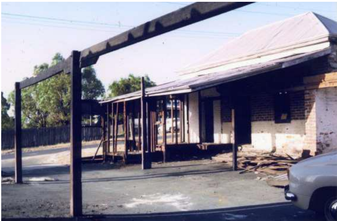
After the fire at the old Terminus Bakery July 1964
