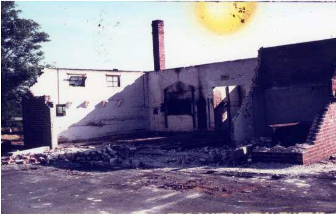
After the fire at the old Terminus Bakery July 1964
